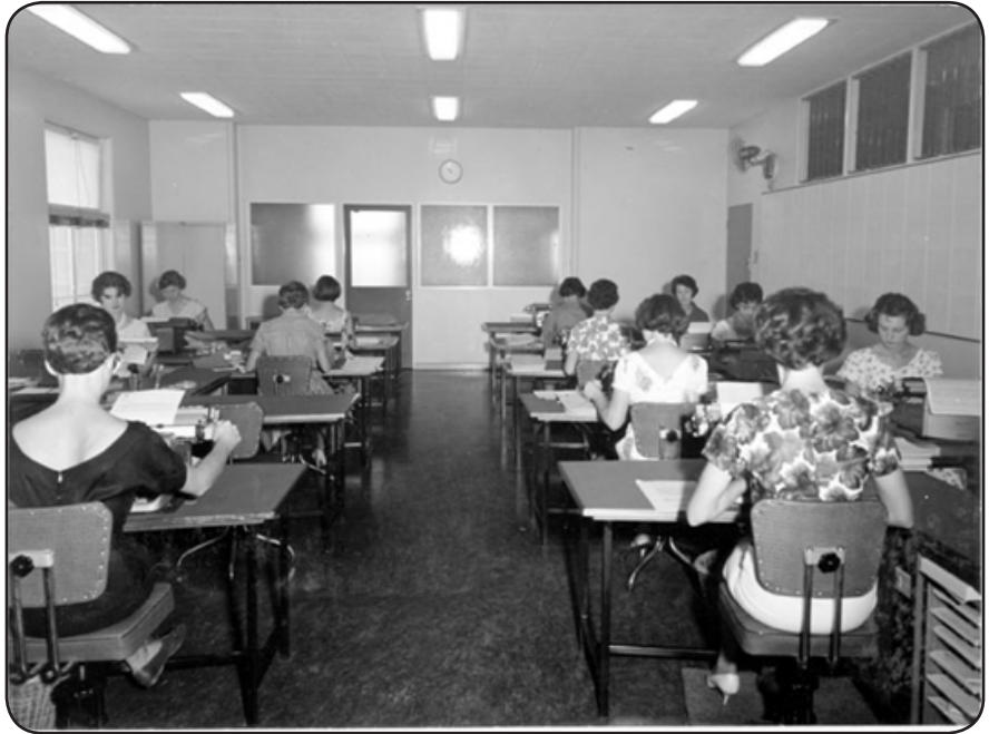
Public Service Commissioner's Department office flooring — Brisbane, March 1962
