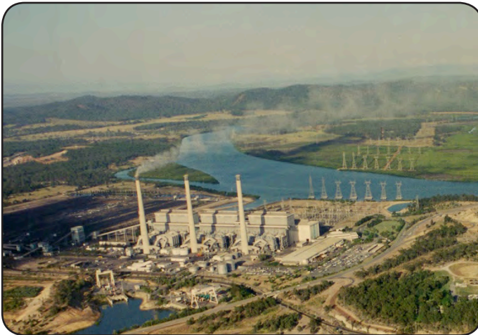
Fig. 3: Gladstone Power Station, early 1990s (GPS collection)
