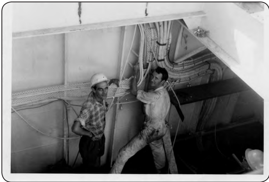
Electricians at work
