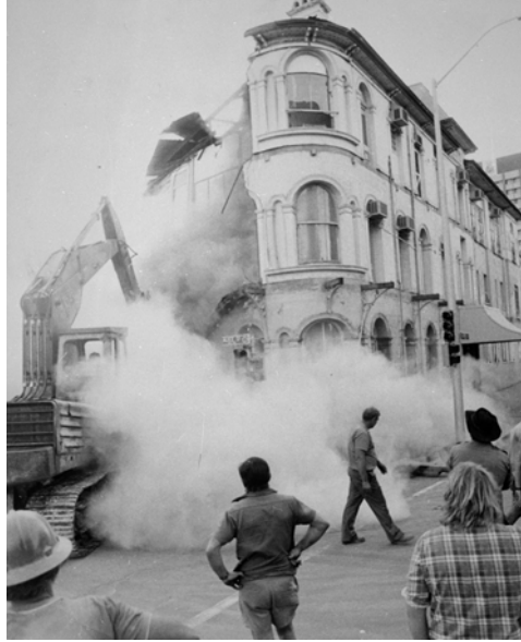
Construction workers watch the demolition of the Bellvue Hotel, Brisbane, April 1979. State Library of Queensland negative number: SLQ 79158.
